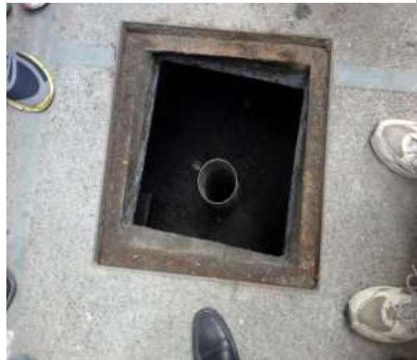
Overflow from Storm drain is directed to Sewer line – in a systematic manner
